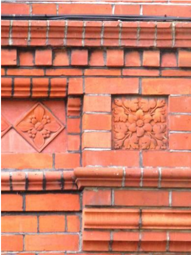
Terra cotta detailing and original timber sash windows with early glass
