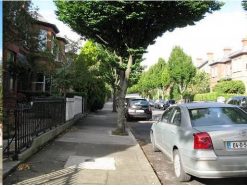
Double height canted bay on Victoria Road
