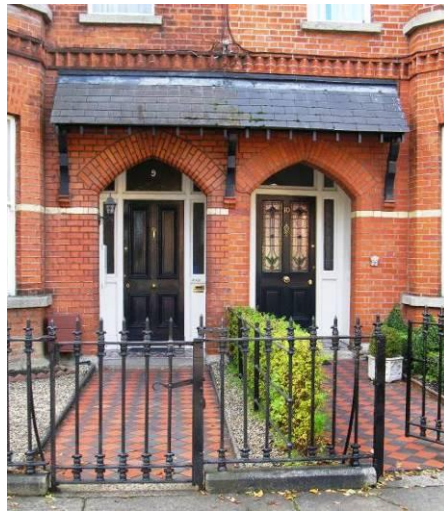
Paired porch entrance doors
