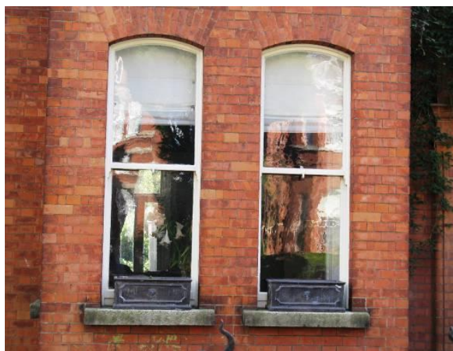
Terra cotta detailing and original timber sash windows with early glass
